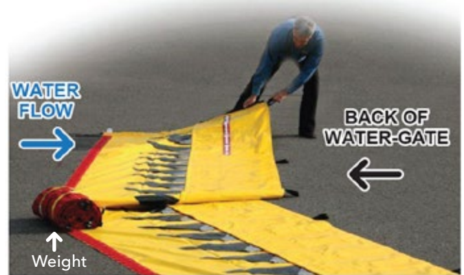
B - Place weights on the front flap of the Water-Gate as a pivot point and turn unit to the desired angle.
